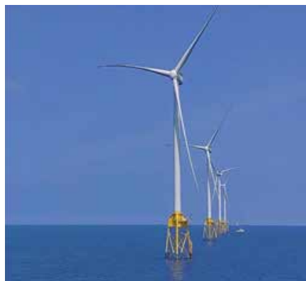
▲ Figure 4-5 Offshore Wind Farm
